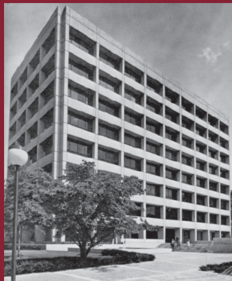
1973: H. William Close Building
